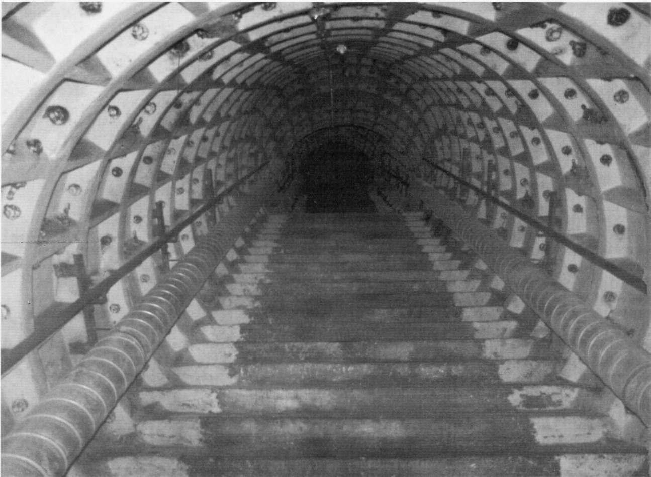
Staircase up to Clapham North station (now blocked) from shelter
